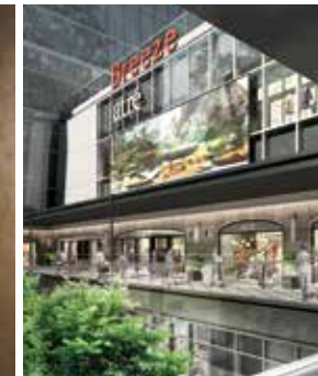
Exterior view of Atre in Breeze Nanshan
