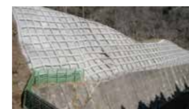
Natural slope protection (spray frame work)
