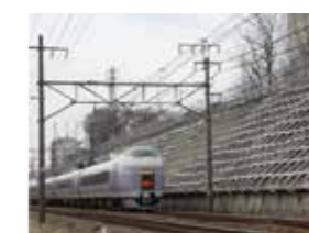
Cutting slope protection (spray frame work)
