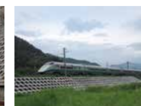
Embankment slope protection (spray frame work)
