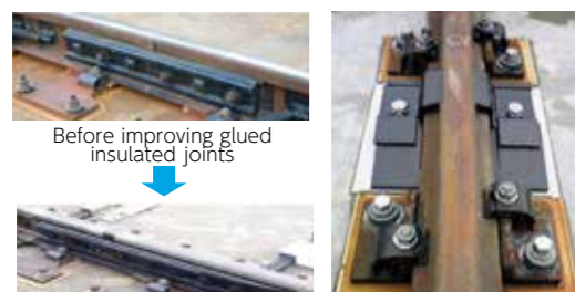
Rail rollover prevention devices
