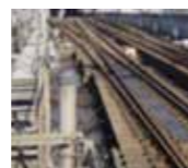
Snow melting mat to prevent point-switching failure
