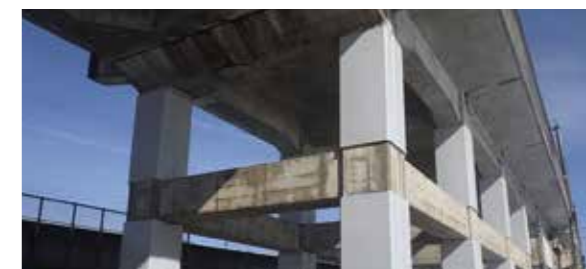
Seismic reinforcement
