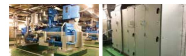
High-efficiency turbo refrigeration and air conditioning units after facility upgrading
