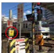
Level crossing alarm system
