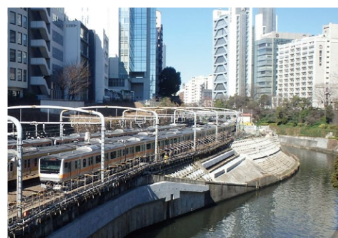
Seismic reinforcement of embankment
