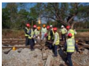
Track maintenance in Myanmar (PC sleeper replacement)
