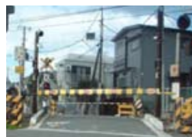
A large crossing gate
