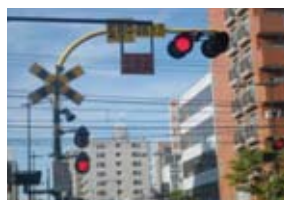
A crossing warning device located in a higher position for better visibility
