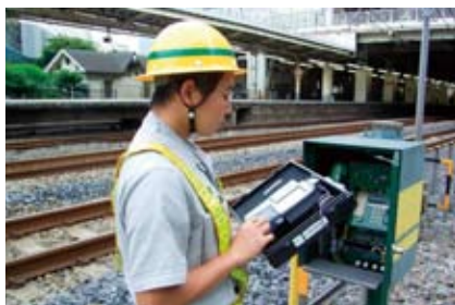
Track closure procedure by a handheld device for maintenance work
