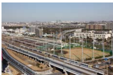
Large-scale solar power generation facility (Keiyo Rolling Stock Center)
