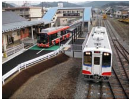
Ofunato line BRT, Sakari Station
