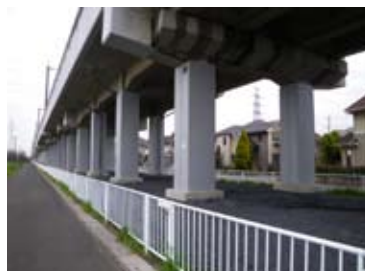
Examples of seismic reinforcement
