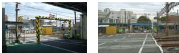
Now-closed Sojiji Temple rail crossing on the Tokaido Line
