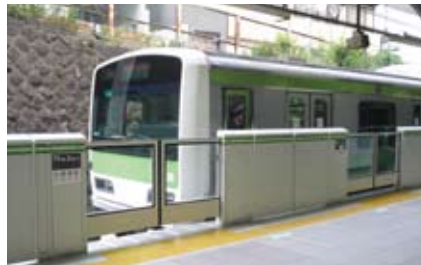
Automatic platform gates on the Yamanote Line
