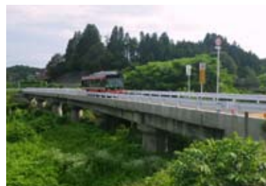
A bus running on a widened railway bridge
