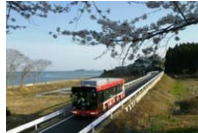
Completed BRT road and a bus running on it
