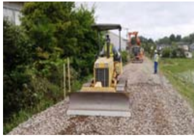
Use of improved ballast as the BRT road bed
