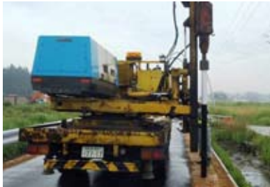
Use of damaged rails as earth retaining piles (driving-in of rails)
