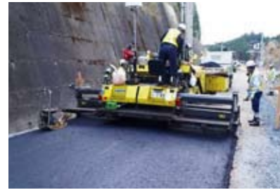
Asphalt paving of BRT road
