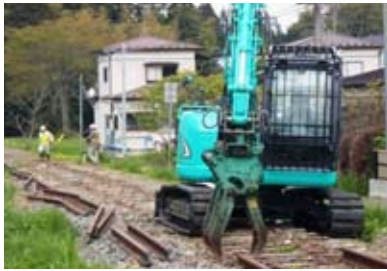
Removal of track materials (rails, ballast, sleepers) in the earthquake-affected area
