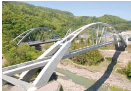
Agatsumagawa Bridge No. 3
