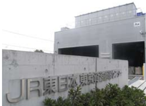
JR East Tokyo Materials Recycling Center
