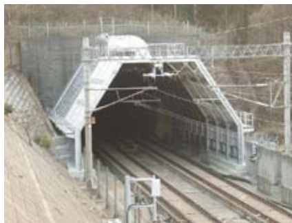
Tunnel hood with a duct
