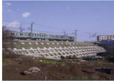
Concrete lattice frame protection work
