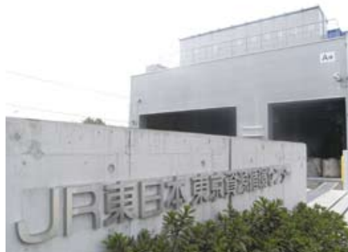
JR East Tokyo Materials Recycling Center
