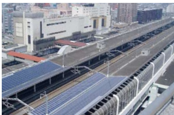
Solar panel installed atop platform roofs at Takasaki station
