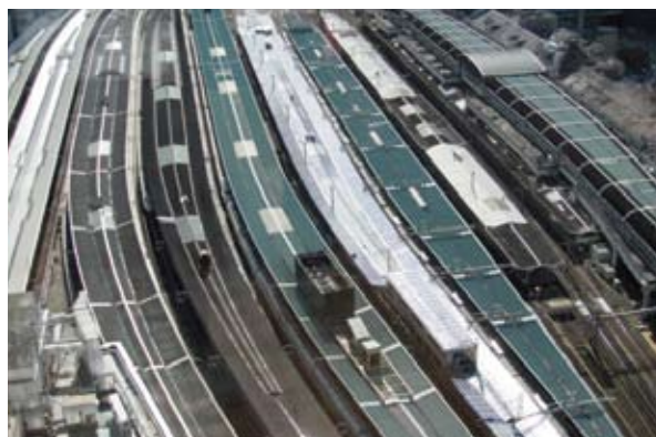
Solar panels installed atop Tokaido Line platforms (Tracks No. 9 and 10) at Tokyo station
