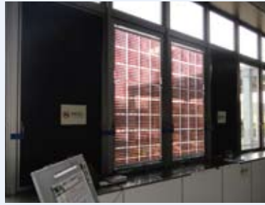
Light transmissive organic thin-film solar cell
