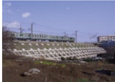
Concrete lattice frame protection work
