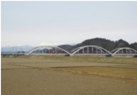
Using continuous concrete arches, the Tenmagawa Bridge, between Kamikitamachi and Ottomo on the Tohoku Main Line, sits in harmony with the mountains and pastoral landscape of Aomori Prefecture and received the 2008 Civil Engineering Design Prize of the Japan Society of Civil Engineers.
