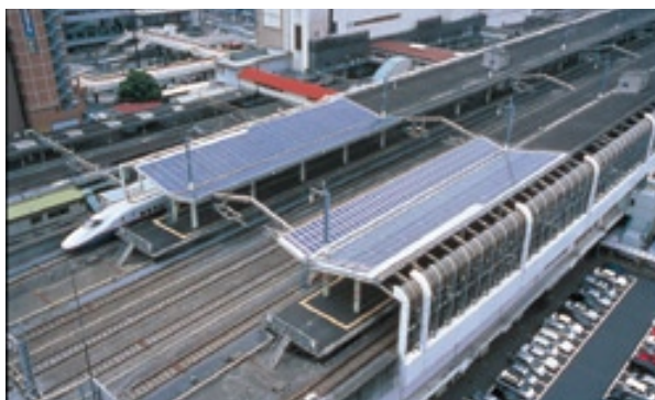
Solar panel installed atop platform roofs at Takasaki station.
