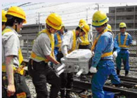
Training on exchanges of motors that move points at turnouts
