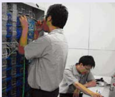
Training on wiring for equipment controlling signal devices
