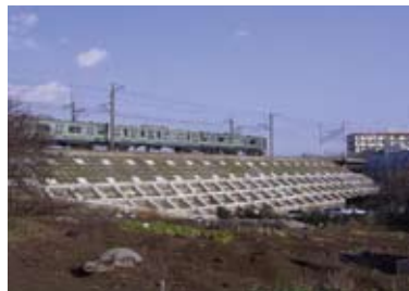
Concrete lattice frame protection work
