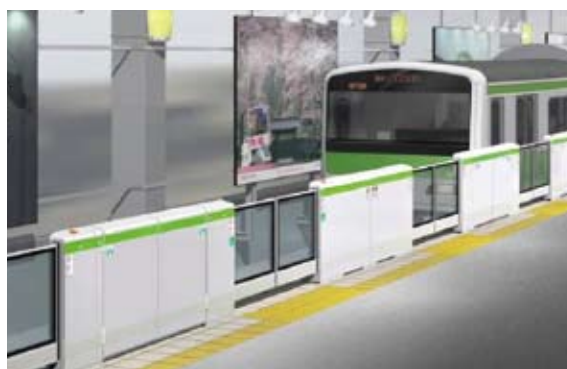
Automatic platform gates on the Yamanote Line (image)
