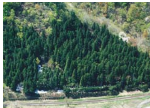
Tenoko No.6 railway forest on the Yonesaka Line (forest to protect against snowslides)
