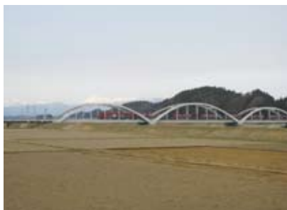
Using continuous concrete arches, the Temmagawa Bridge, between Kamikitamachi and Ottomo on the Tohoku Main Line, sits in harmony with the mountains and pastoral landscape of Aomori Prefecture and received the 2008 Civil Engineering Design Prize of the Japan Society of Civil Engineers.
