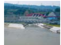
Shinanogawa Hydropower station producing clean energy without emitting CO 2 .
