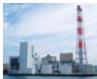
At Kawasaki thermal station kerosene was replaced with natural gas to run No. 3 generation unit in June 2006.
