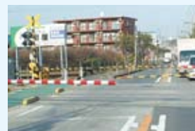
A red and white large crossing gate, to improve visibility and deter careless crossing of railway tracks
