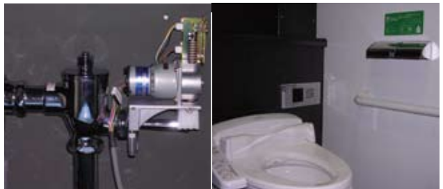
Automatic water flow controller for toilets (BT-Crab)—reduces toilet water consumption by 50%
