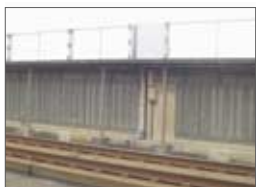
Installing sound-absorbing panels
