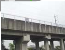
Raising the height of soundproof walls
