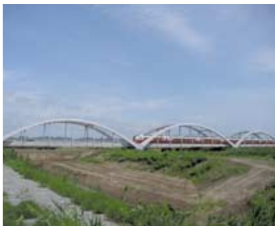
The bridge over River Tenma between Kamikita-cho and Ottomo on Tohoku Main Line, where serial concrete arch design is adopted in an effort to create harmony with the beautiful scenery of the mountains of Aomori.
