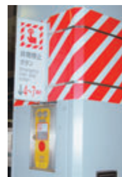
Train drivers are notified of any danger through emergency stop buttons placed on platform columns.
