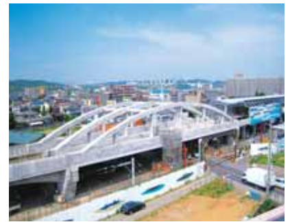
The height of the front and back guiderails of Yanoguchi Bridge, serving the Nambu Line, corresponds to that of the main beams to give an appearance of continuity. This is Japan's first Langer truss bridge with three main beams for a double track railway.
