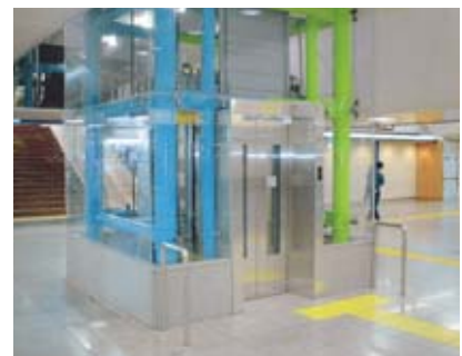
We are installing elevators to eliminate barriers to mobility.
