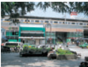
Above: Before refurbishing Below: After refurbishing Asagaya Station on the Chuo Line was refurbished as part of our Station Renaissance program (see page13). The project focused on harmonizing with surroundings.
