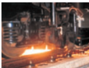
Smoothing rail unevenness caused by train operation
