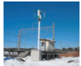
Windmills on wind power generators at Gosawa Station on the Tsugaru Line rotate in any wind direction
