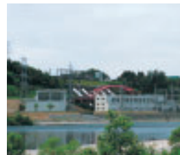
Shinano River hydroelectric plants emit zero CO 2 or other harmful gases
