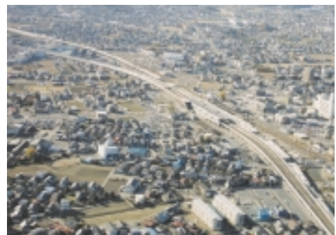
Continuous overhead crossing
