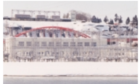
Shinano River Power Plant
