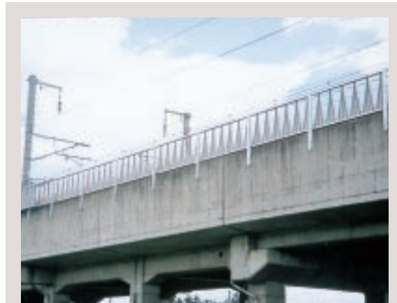
Triangular-peaked soundproofing device minimizes noise while preserving the view from railcar windows.
