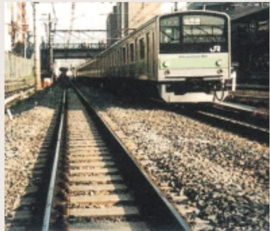
"TC-type low-maintenance roadbed," introduced to reduce labor spent in maintenance work
