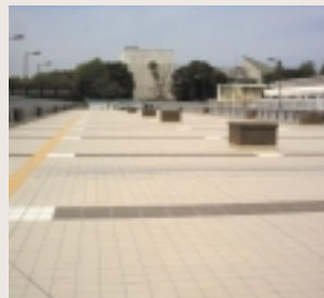
Recycled paving tiles made from glass bottles (train passageway at Ueno Station)
