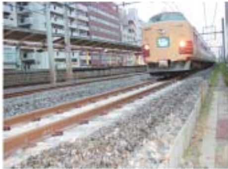
Fig. 20: Test Tracks Laid on an Operational Line
