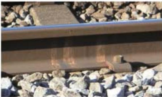
Fig. 2: External Appearance of a Welded Part of a Rail (as seen from the side)
