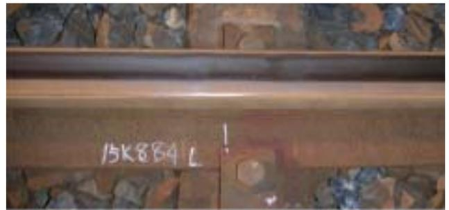
Fig. 3: External Appearance of a Welded Part of a Rail (as seen from above)
