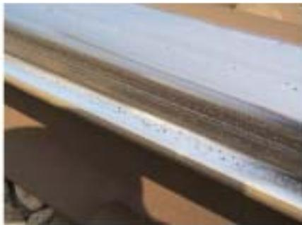
Fig. 8: Rail in which Wear has Progressed
