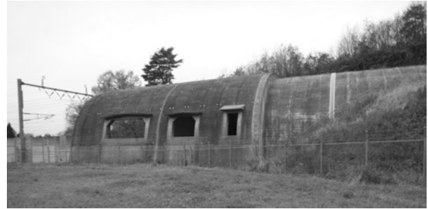
Fig. 3 Tunnel Hood Slits
