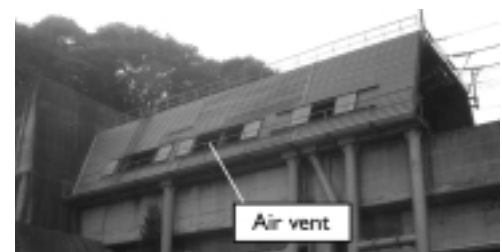
Fig. 2 Hood at tunnel entrance
