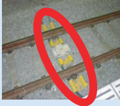
Protective pipe installation (approximately 1,400 locations)
