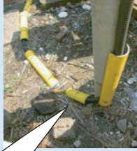
Installation of covers to prevent accidental severance (approximately 31,500 locations)
