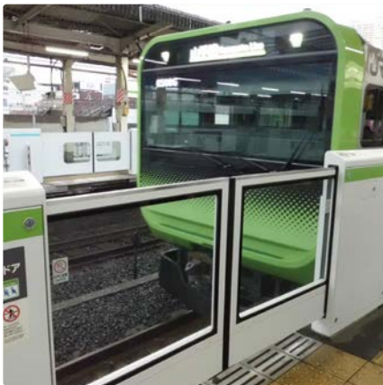
Automatic platform gates
