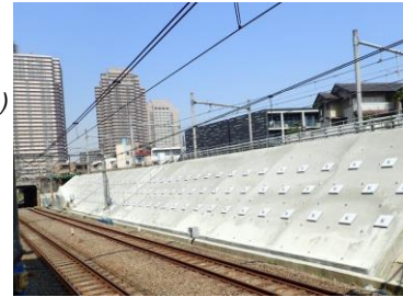
Seismic reinforcement of embankments
