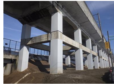
Seismic reinforcement of viaduct columns
