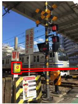
Safety measure for railway crossing
