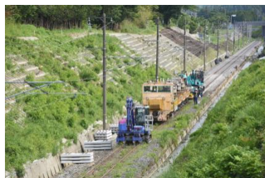
Earthquake recovery (Joban Line)
