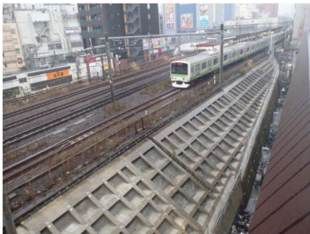
Seismic reinforcement of embankments
