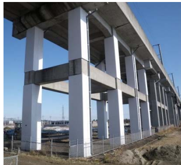
Seismic reinforcement of viaduct columns
