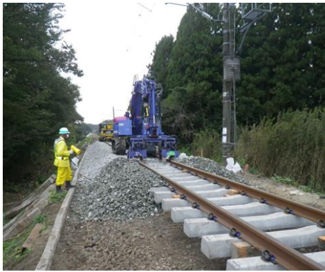
Restore conventional lines damaged by the Great East Japan Earthquake (Joban Line)
