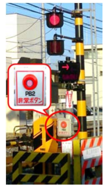
Safety measure for railway crossing
