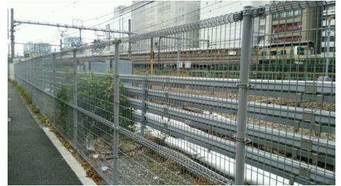
Strengthening railway-related security (fence installation)
