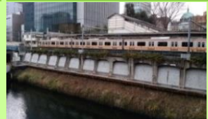
Seismic reinforcement of bridge piers
