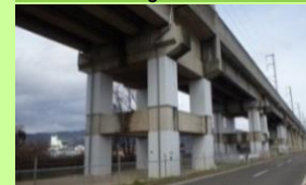
Seismic reinforcement of elevated bridge columns
