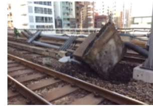
Collapse of electrical pole on Kanda–Akihabara segment of Yamanote Line
