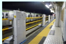
Vertical-motion automatic platform gates at Haijima Station
