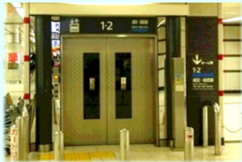
Increased installation of elevators in Narita Airport Station
