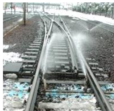
Measures to prevent railroad switch malfunctions
