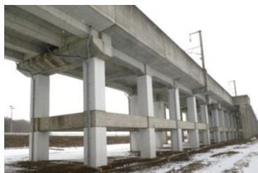
Seismic reinforcement of viaduct columns
