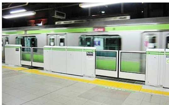
Automatic platform gates
