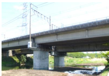
Seismic reinforcement of bridge piers
