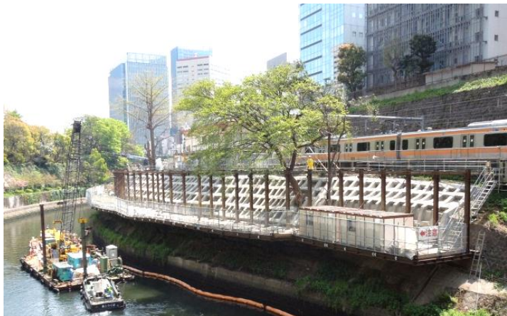
Seismic reinforcement of embankments
