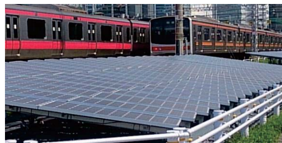
Solar power generation equipment
