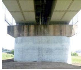
Seismic reinforcement of bridge piers
