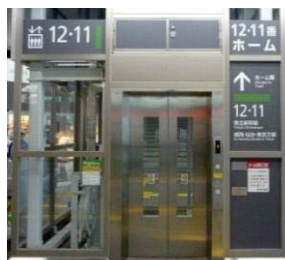
Elevators at stations
