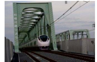
Tone River bridge
