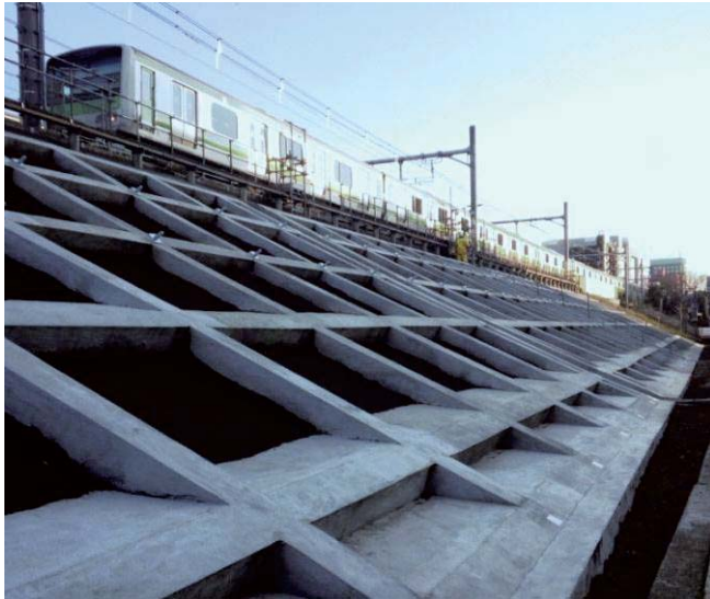
Seismic reinforcement of embankments
