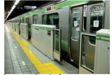
Automatic platform gates on the Yamanote Line
