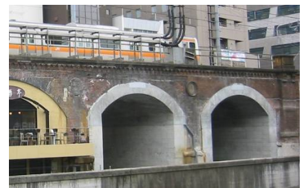
Seismic reinforcement of brick arch viaducts
