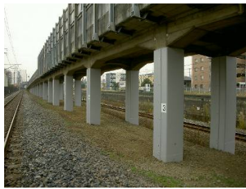
Seismic reinforcement of viaduct columns
