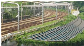
Seismic reinforcement of embankments
