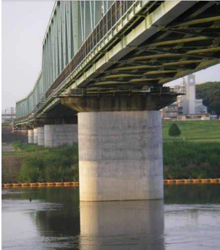
Seismic reinforcement of bridge piers
