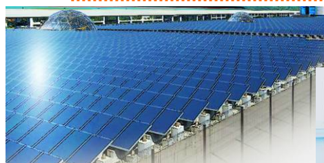
Solar power generation equipment
