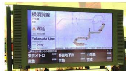
Installation of emergency information displays
