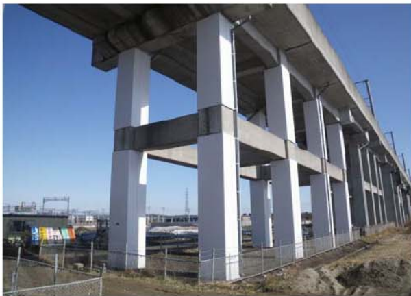
Seismic reinforcement of viaduct columns
