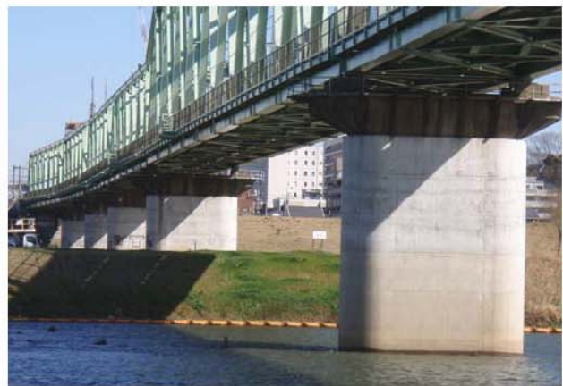
Seismic reinforcement of bridge piers
