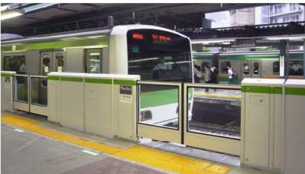
Installation of platform doors on Yamanote Line
