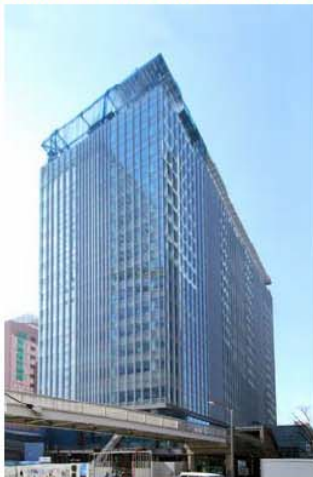
JR South Shinjuku Building
